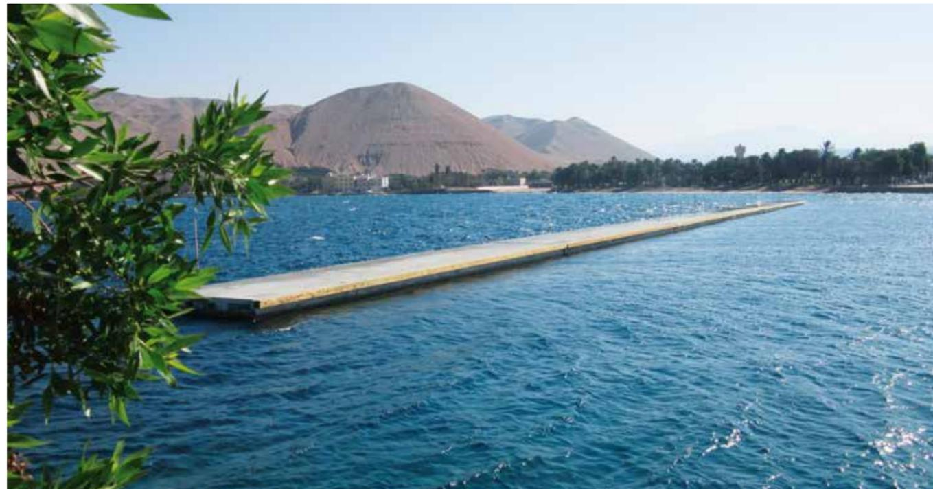
rotational polyethylene with expanded polystyrene core, varies according to the specific conditions of use.
