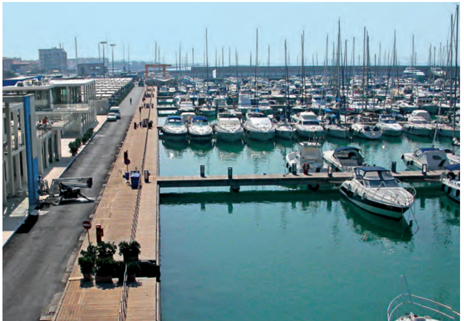
Cantilever fixed quay 3.20 m wide
