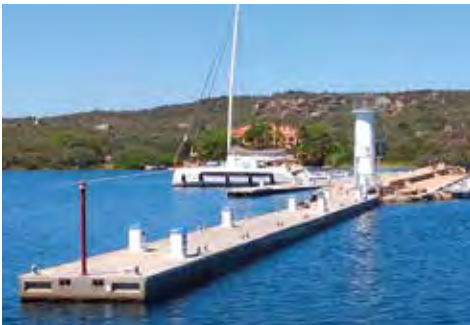
Pianottoli - France: floating breakwater for the Municipal port in the Bay of Figari
